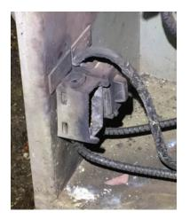
A jointer checking supplies in an LV distribution board decided to remove a street light cut-out fuse from its holder as there had been reports of street lights flickering in the area.
