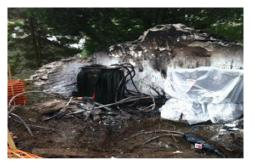
The investigation into the incident identified the most likely cause of the switchboard failure was due to contact pitting, incorrect contact alignment between the fixed and moving contacts on the switch fuse, and the rising busbar being out of its correct vertical plain leading to local overheating and thermal runaway. The previous plant maintenance policy did not require checking of the contact alignment.
