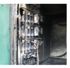
Subsequent investigation revealed that the LV board at the substation had disruptively failed whilst the operative was carrying out an operation to remove fuses on the LV board to isolate a faulty circuit for the jointer to commence work.
